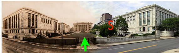
S - Building C security desk E - entrance to Seeley G Mudd o - Rm 130
